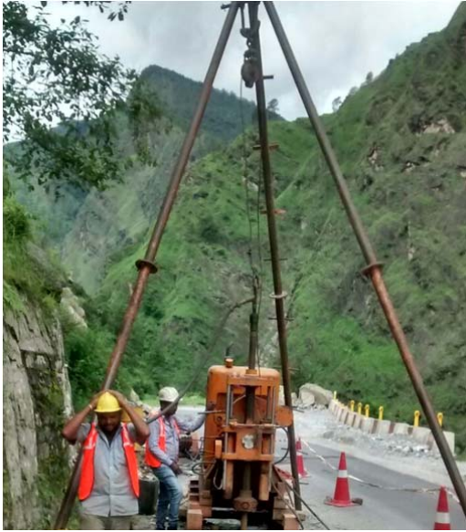
Fig. 2 Borehole drilling in progress
