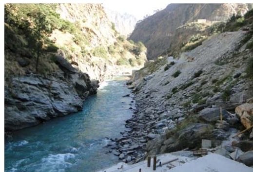
Fig. 8 Eroded River Bank
